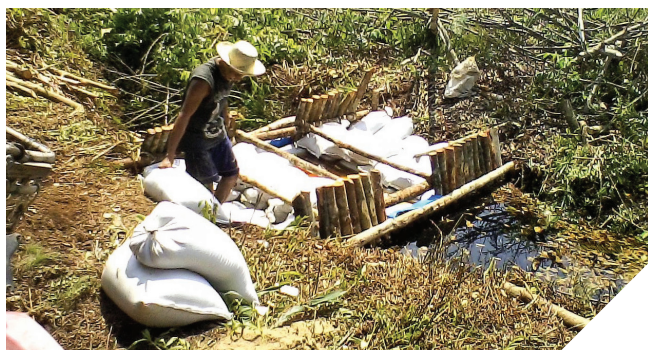
A glimpse of the canal block construction process.
