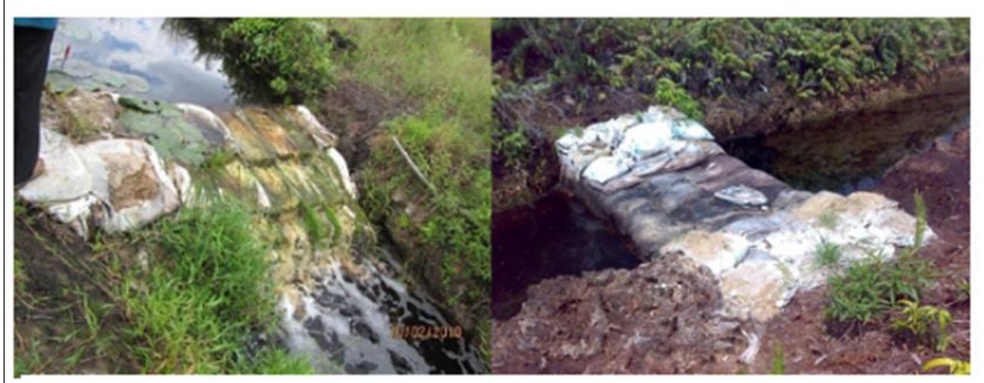
Figure 10. Types of Soilbags Dam (Photo: Ng Kok Seng, 2011)
