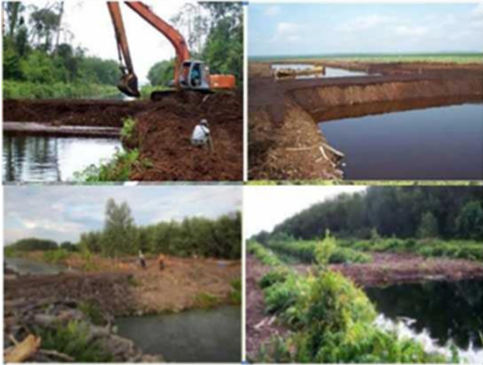
Figure 11. Example of compacted peat canal blocking (Photo: Deltares)
