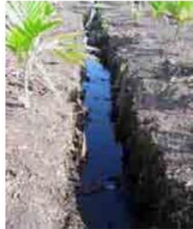
Ditch on Simpang Kiri village (Sumatera) (YRN – ccfpi.doc)
